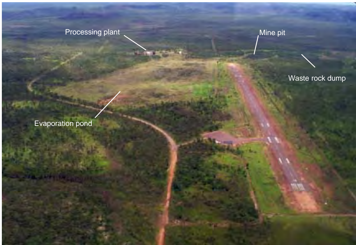
Figure 2 Nabarlek mine site features and the affected streams (Top). Aerial photograph of Nabarlek taken January 1999 (Bottom).
