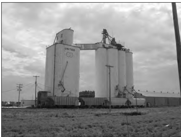
Grain Elevator, Hordville (HM04-023).
